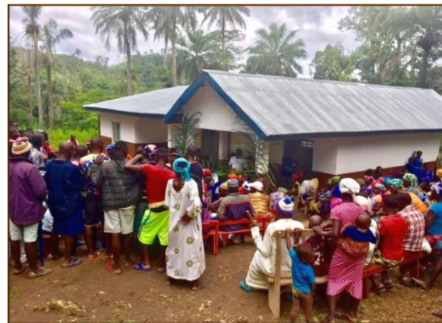
Above: The first stage of the Maternal and Child Health Post is complete. S4LA is continuing to help improve the facilities, extend the basic services and support community health.
