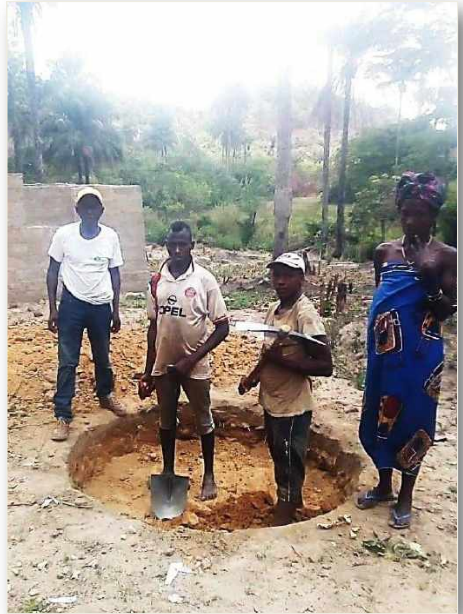
Working began on the clinic well approx 18 months ago.
